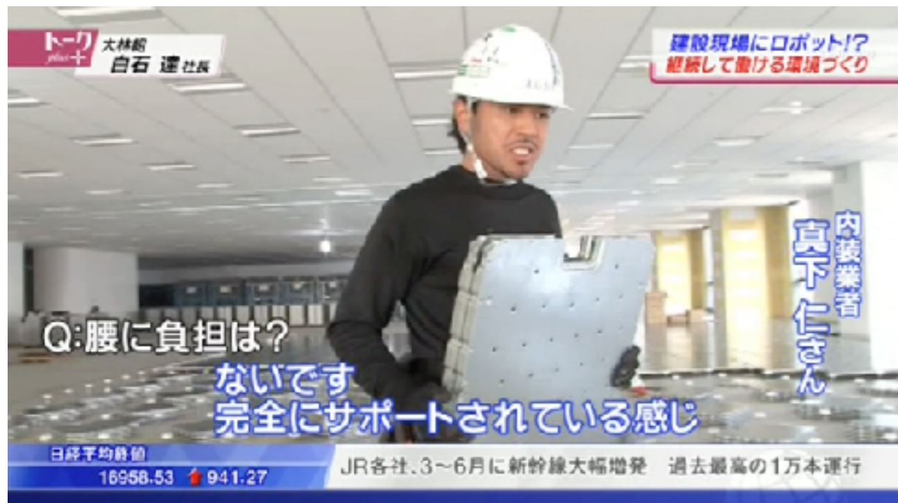
【Construction】 (Obayashi : Laying OA Panels)
