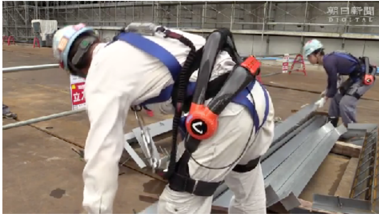
【Construction】 (Daiwa House: Carrying loads)
