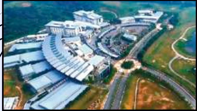
PERKESO - REHABILITATION CENTRE MELALA (Malaysia)
